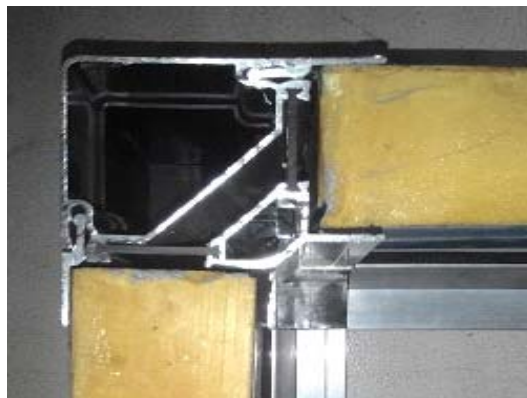
TB1 Frame Profile Cross Section
